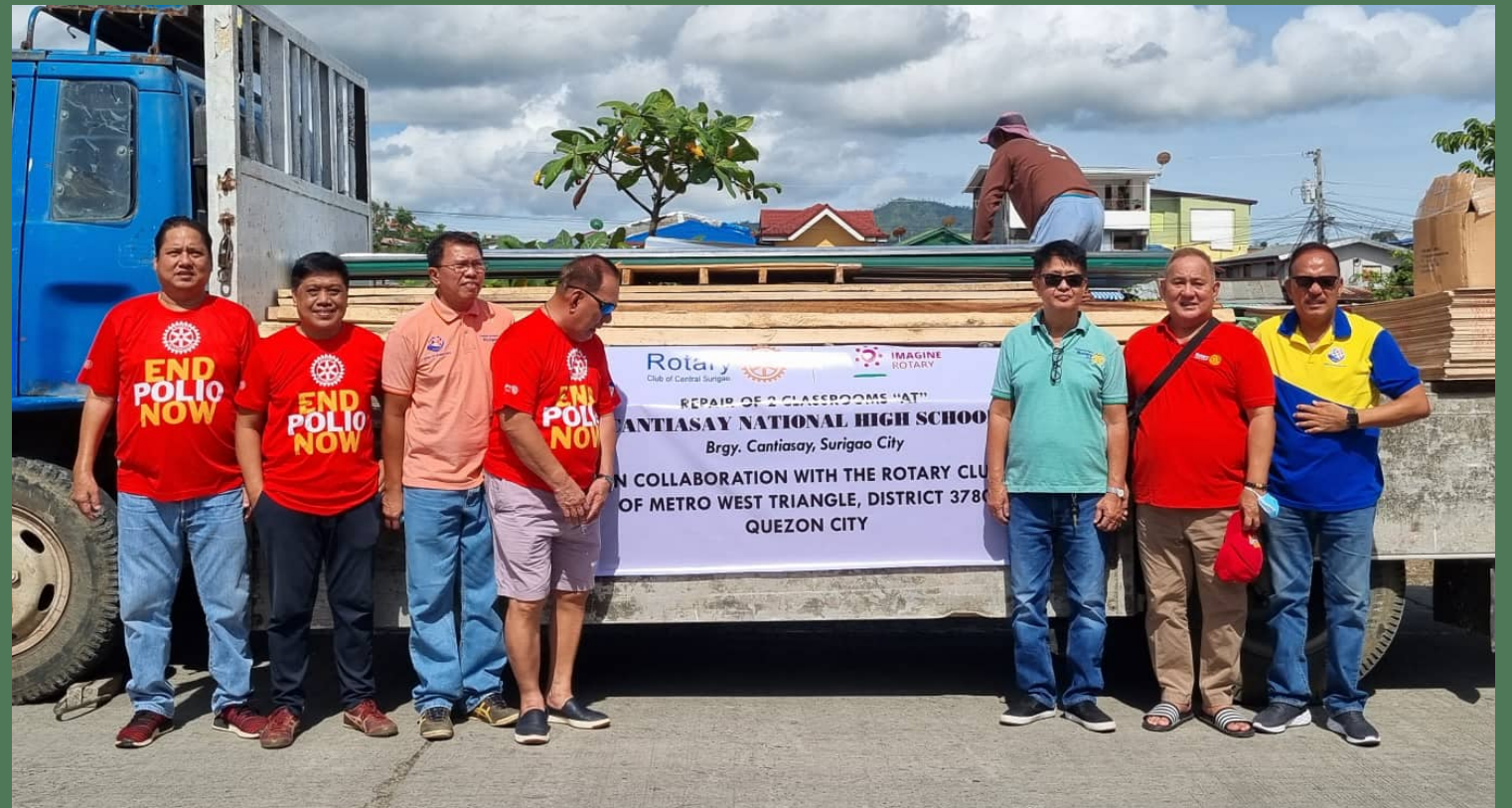
Repair of Classrooms at Cantiasay National High School
